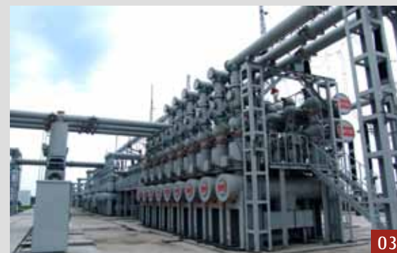
01: 550kV HGIS at Shenzhen \pm 800 kV Yunguang HVDC Converter Substation,China 02: 330kV Dead Tank Circuit Breaker at Hancheng Substation, China 03: 363kV GIS at Shaanxi Weinan Power Substation,China
