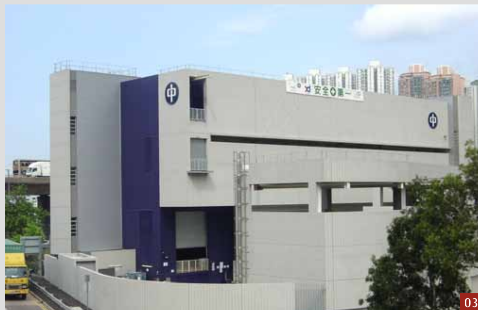
01、02&03: View of CLP New Hoi Shing substation
