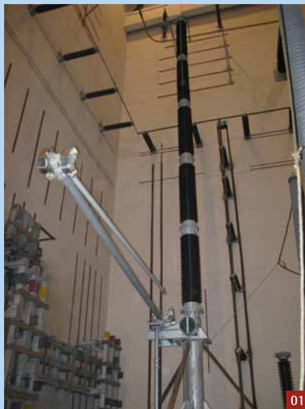
01: 1100kV Earth Switch under installation
