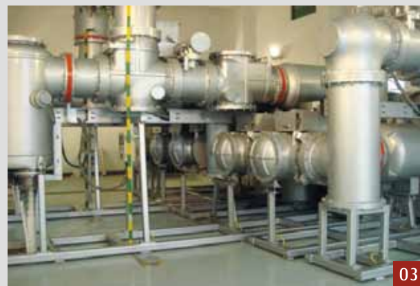
01: 132kV GIS in Mai Po Substation, Hongkong 02: 132kV GIS in Yiu Wing Street Substation, Hongkong 03: 126kV Compact GIS at Changzhou Substation, China 04: 72.5kV GIS for Singapore Power Grid
