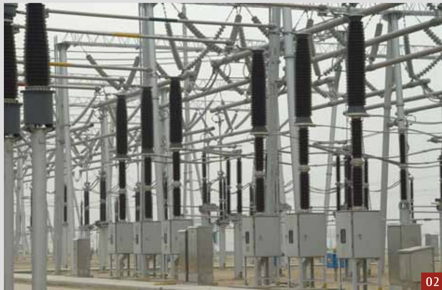
01: 252kV Live Tank Circuit Breaker under installation 02: Commissioning of 252kV Live Tank Circuit Breaker
