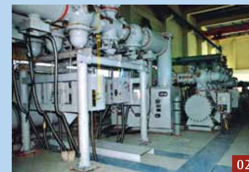
01: 252kV GIS at Shanghai Wanrong Power Station,China 02: 252kV GIS for Pakistan project 03: 252kV Compact GIS
