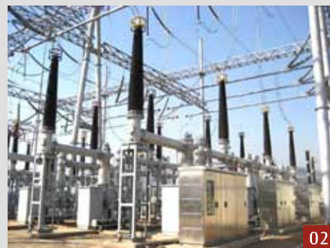
01: 550kV HGIS at Shenzhen \pm 800 kV Yunguang HVDC Converter Substation,China 02: 330kV Dead Tank Circuit Breaker at Hancheng Substation, China 03: 363kV GIS at Shaanxi Weinan Power Substation,China
